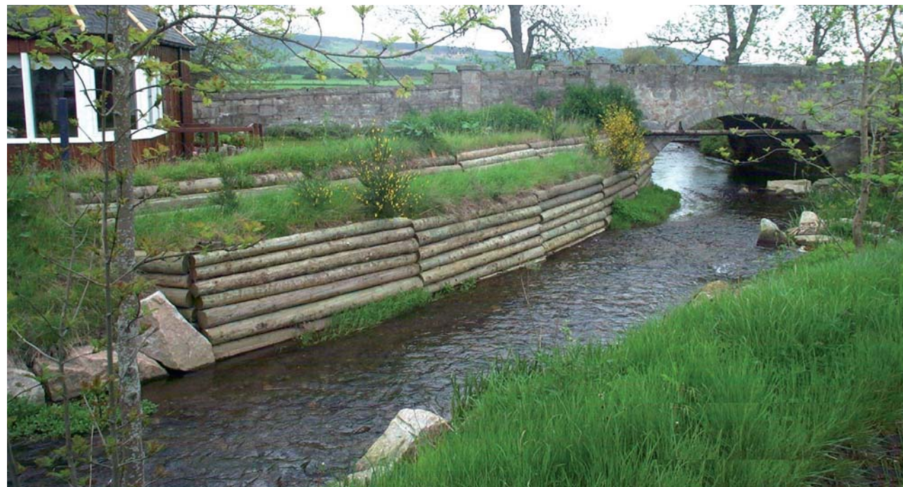
'Soft' bank engineering work (Aberdeenshire Council)
